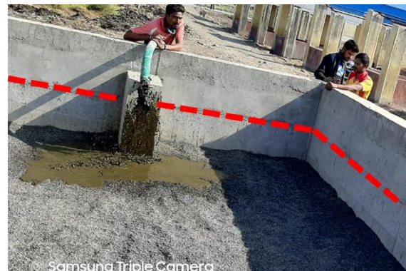
Figure 6 Sludge to be filled up till red marking Source: C-WAS
