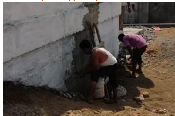
Figure 14 Carrying out annual painting works Source: Khopoli FSTP, (C-WAS)
