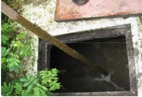
Figure 11: Checking sludge levels
