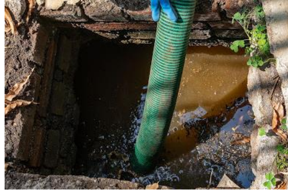
Figure 12 Desludging first chamber of ABR unit
