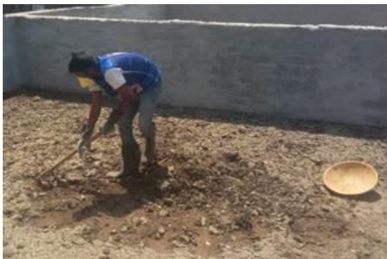
Figure 7: Removing dried sludge using shovel Source: Khopoli FSTP (C-WAS)
