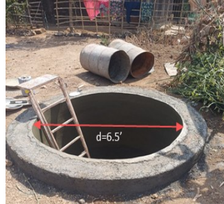
Brick Masonry Underground Storage Tank, Mahagaon
