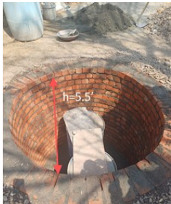
Brick Masonry Underground Storage Tank, Mahagaon
