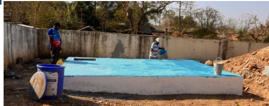
Underground Rectangular Tank with RCC slab; Piping and handover process to be done before monsoon
