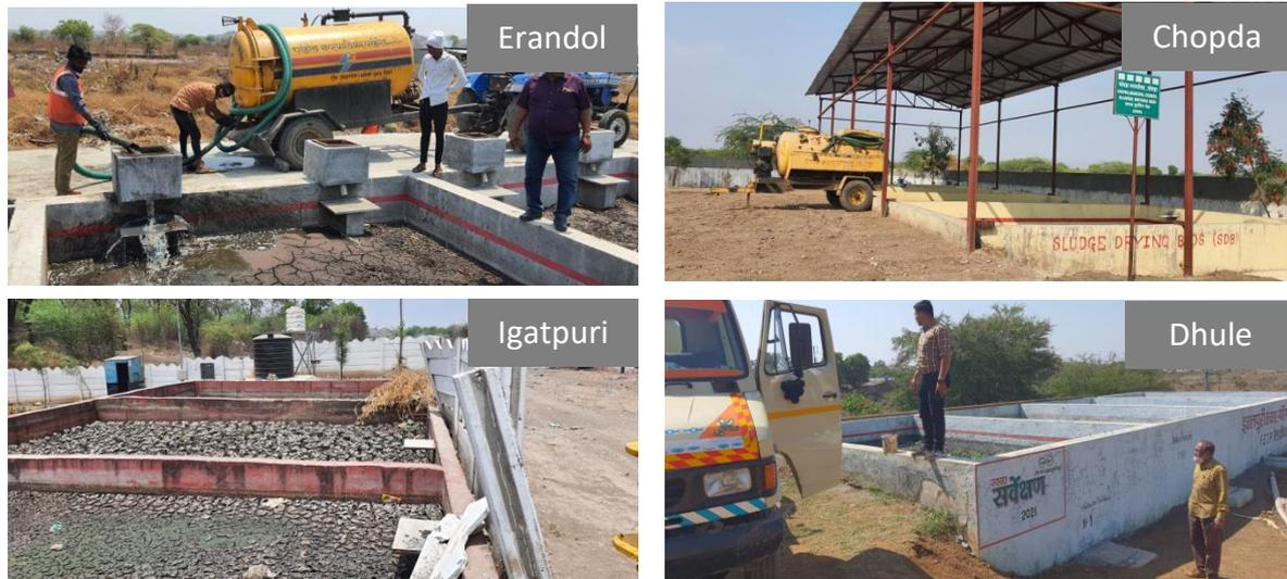
Figure 4: Sludge drying beds in Erandol, Igatpuri, Chopda and Dhule
