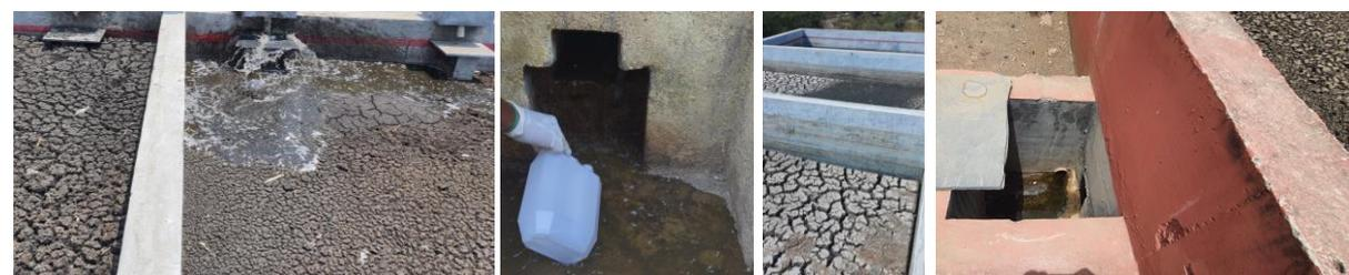
Figure 7: Collection of dried sludge at FSTPs in Erandol, Igatpuri, Chopda and Dhule (From left to right)
