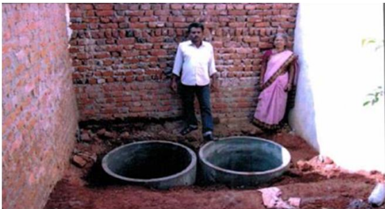
IHHT constructed through Vipanchi Area level federation
