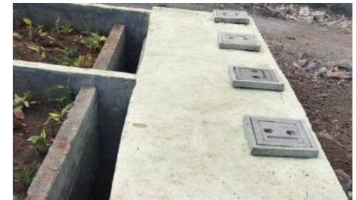
Bhor Anaerobic baffle reactor + PGF
