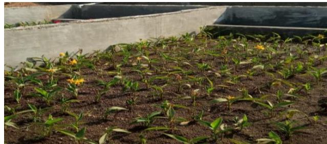
Peth Planted gravel filter
