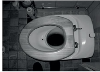
Figure B.4 — Sitting and squatting types of urine diverting dry toilets (UDDT)
