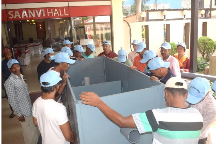
Training for Masons on Construction of Standard Septic Tanks
