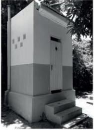
Figure B.3 — Ventilated improved pit latrine/fossa alterna
