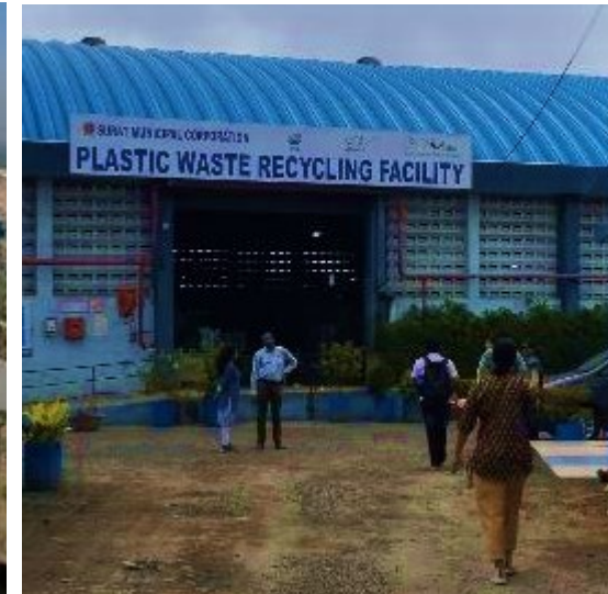
Plastic Waste Recycle Facility
