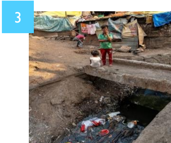
3 Upgradation of open surface drains to closed drains for storm water drainage
