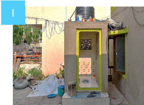
1 Construction of individual toilets (to achieve 90-95% coverage)
