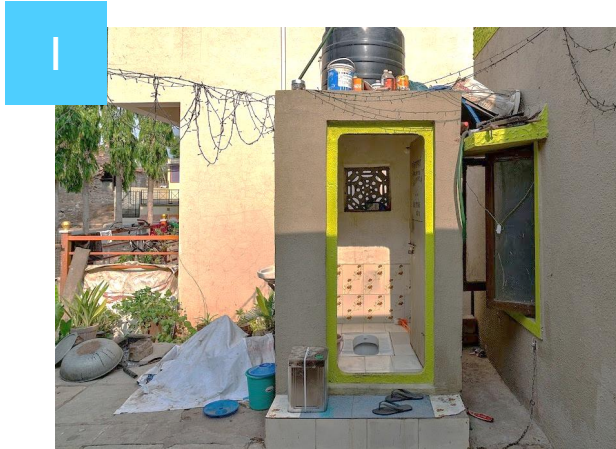
Construction of individual toilets (to achieve 90-95% coverage)
