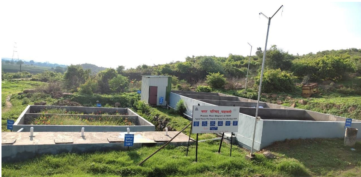
Figure 3 FSTP at Bhadrawati Municipal Council
