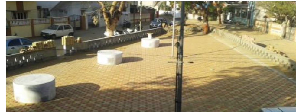
Flood control through GW recharge for a housing colony
