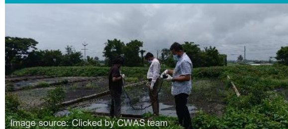
Quantification at sludge drying bed of STP
