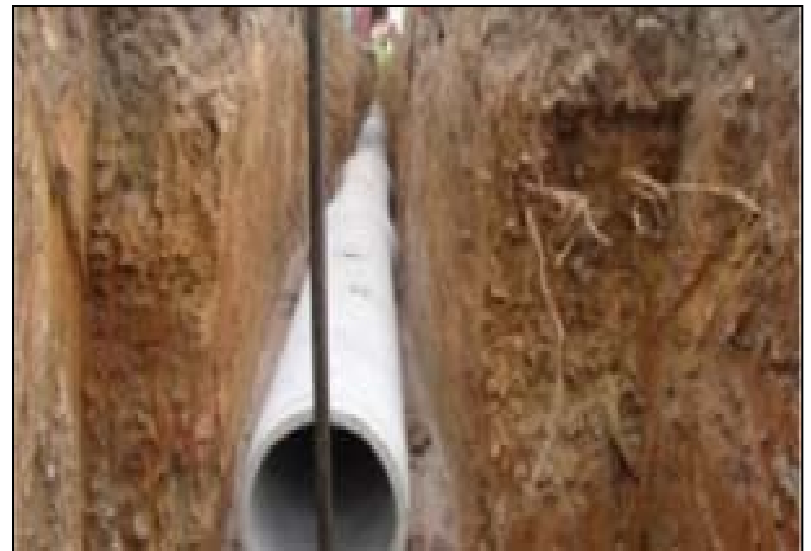
Laying of sewer
