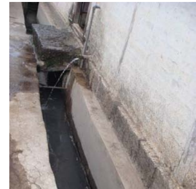
Clean drains in Wai Municipality that carry storm water and grey water
