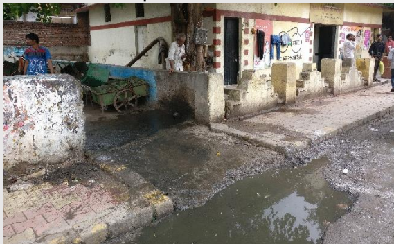
Open Drainages near Astodia Gate
