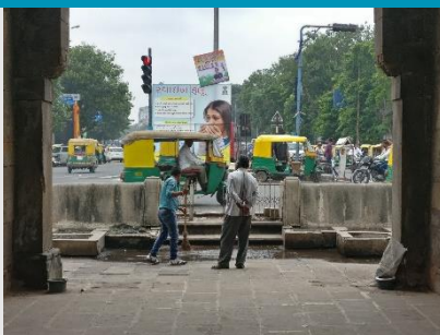
Water Logging due to rise in Road level
