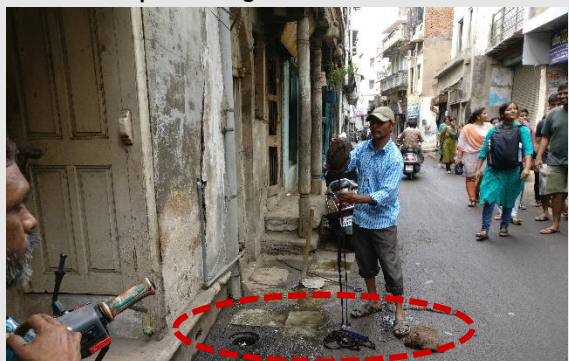
Manual Process of Cleaning Old Drainages
