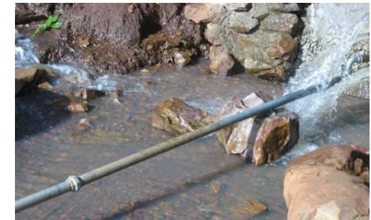
Unaccounted water use
