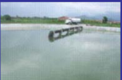
Sludge Lagoon System Completed : 1 Nos
