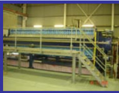
Filter Press 83 units
