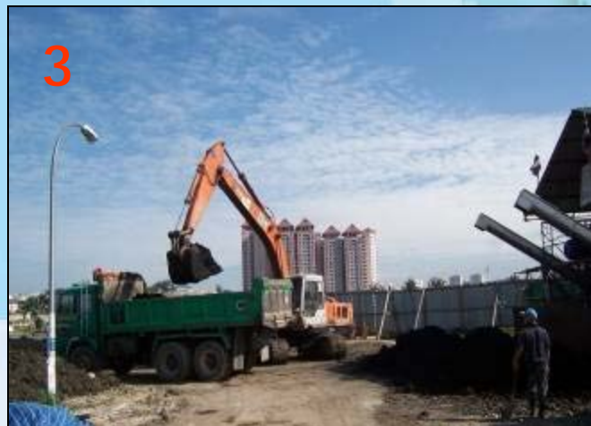
Dried Sludge to be Disposed Off to an approved site
