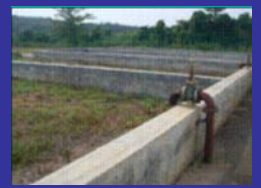
Drying Beds Completed : 3 Nos
