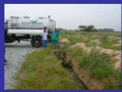
Trenching System Completed : 25 Nos
