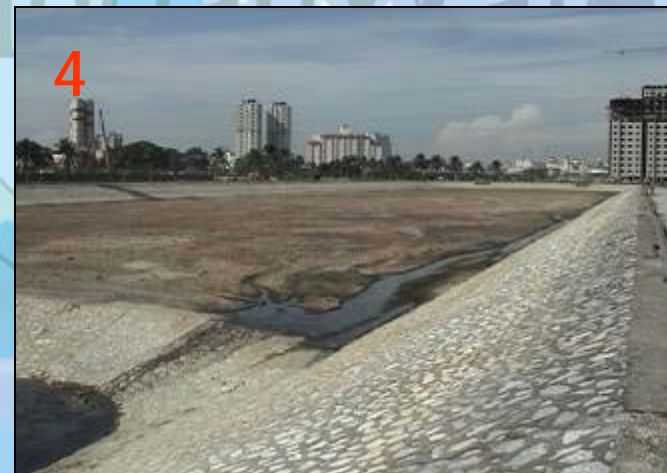
View of Pond after completion of Desludging Exercise
