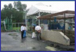
Mechanised Dewatering Unit Completed : 23 Nos
