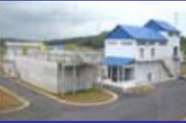
Dedicated Centralised Sludge Treatment Completed : 8 Nos
