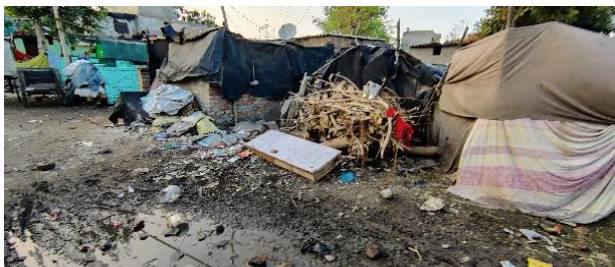
Dilapidated housing without toilet
