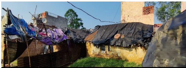
Housing in slum with no space to construct toilet
