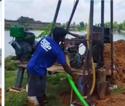
04. Fixing of shaft for drilling of bore well (approximately 7" dia & 2' deep)
