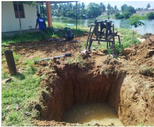
01 Digging a pit for circulation of water while drilling the filter borewell hole
