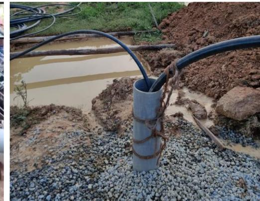
08. Filling the gap with Jelly. Pumping out Muddy water with Air compressor
