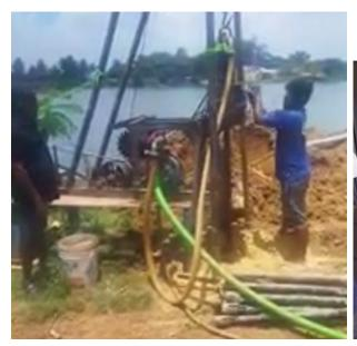
06. <u>3 feet rod will be added one after</u> the other till they get the hard rock 03. <u>4 rods will be arranged</u> <u>for balancing & to place</u> <u>drilling equipment</u> 04. Fixing of shaft for drilling of bore well (approximately 7" <u>dia & 2' deep</u>)
