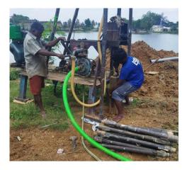
05. Green Pipe is the inlet from storage tank. Black and yellow hose pipe is outlet from drilling machine to circulate the water
