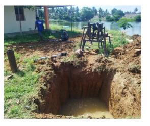
01 Digging a pit for circulation of water while drilling the filter borewell hole
