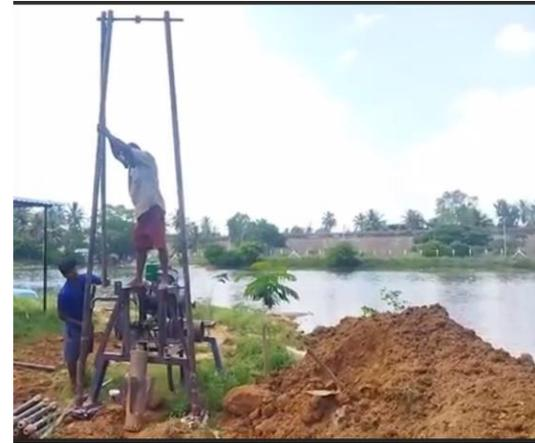
03. 4 rods will be arranged for balancing & to place drilling equipment
