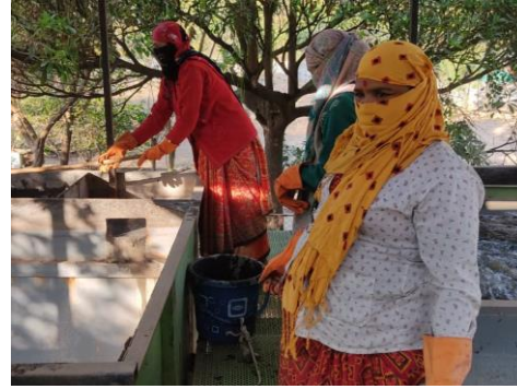
O&M of Grey water treatment plant in Sinnar .
