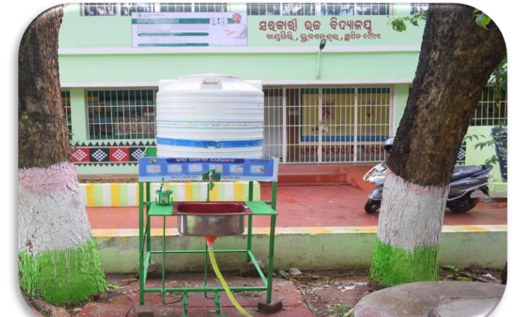
Handwashing station in front of School, Ward 63
