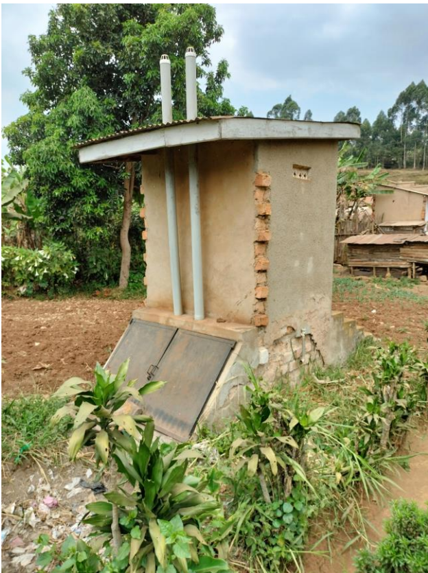
1% - constructing elevated ecosan latrine
