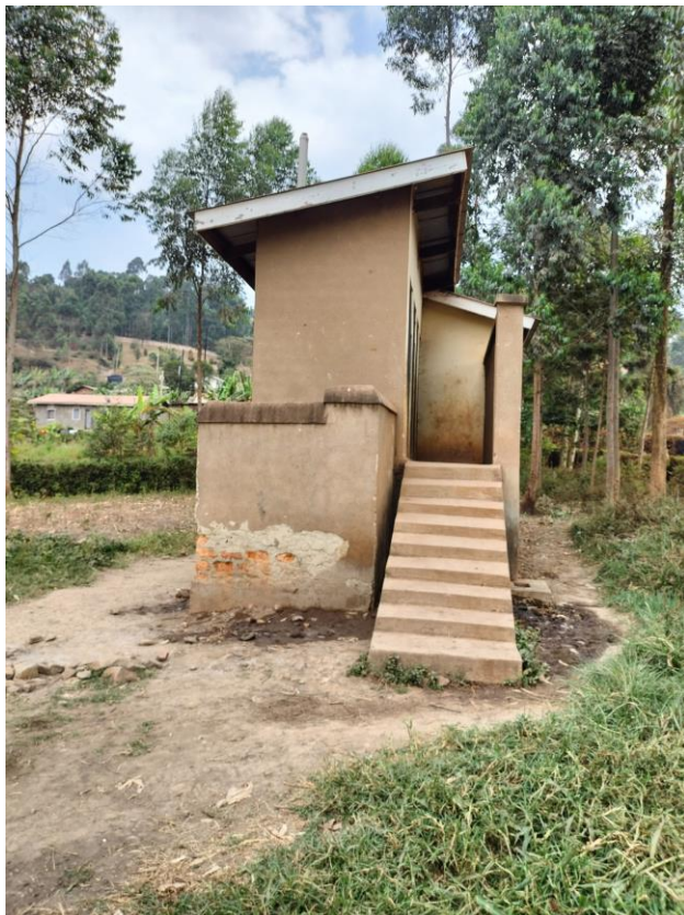
35% - construction of step latrine
