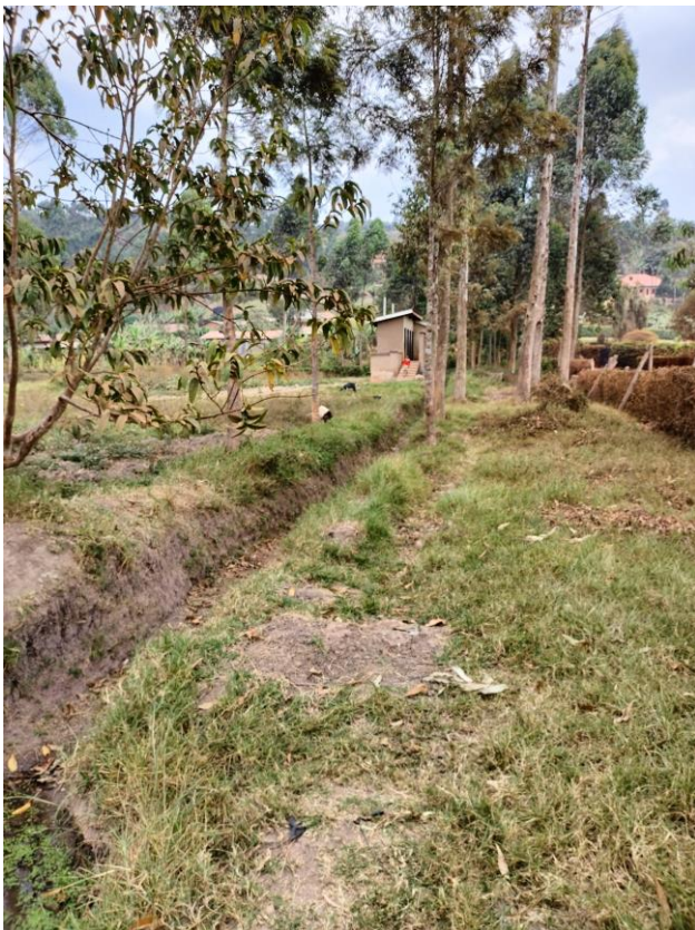
55% - establishment of diversion channels
