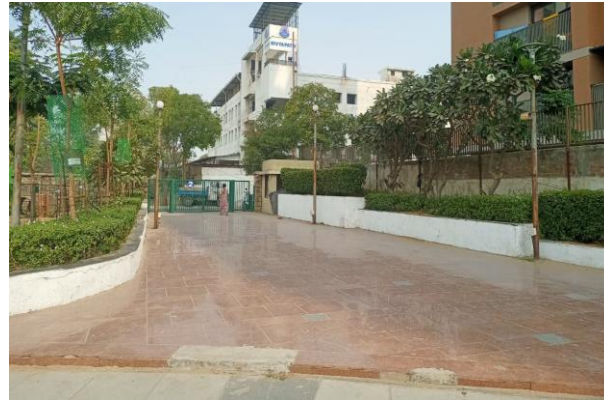
Concrete edges around the lake
