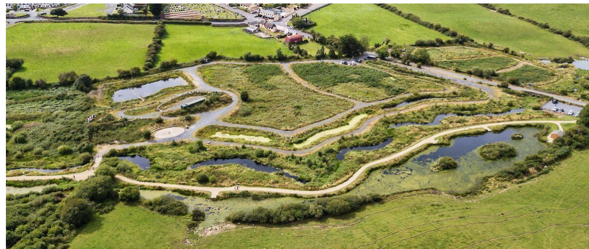
Figure 15: A Constructed Wetland that Includes Different Modules for Filtration
